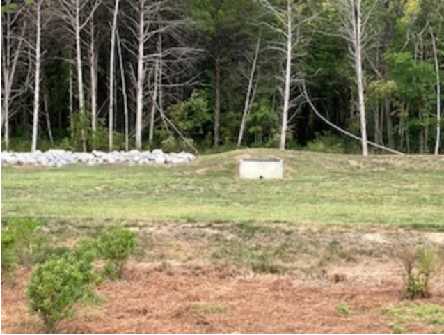
Bio Retention SCM at bathrooms at Golden Bear Park
